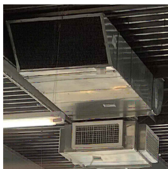
EXAMPLE PHOTO OF HOW THE HVAC SYSTEM IS INSTALLED.
